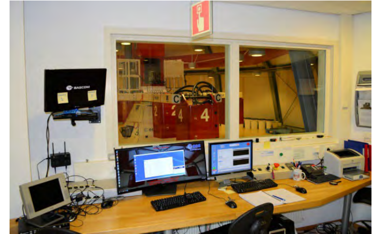
LDC control room
