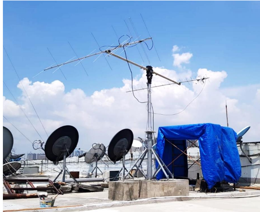
Antenna Installed – 13 September 2022
