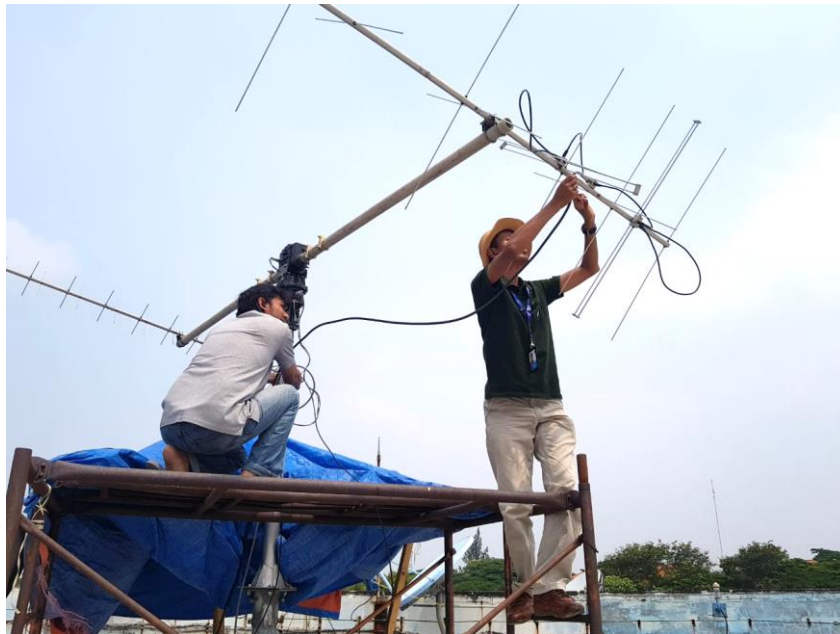
Antenna Construction – 5 September 2022
