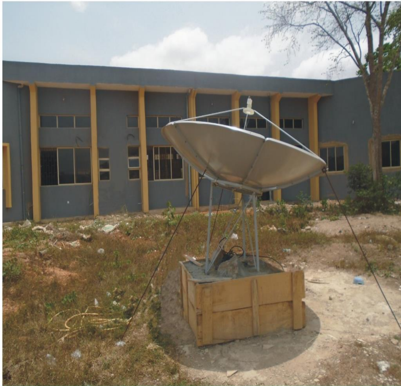
On-going EUMetcast C-Band installation at ARCSSTE-E Space Museum, OAU, Ile-Ife.
