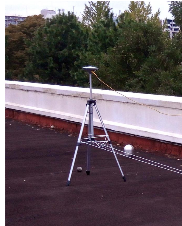
Temporary base station
