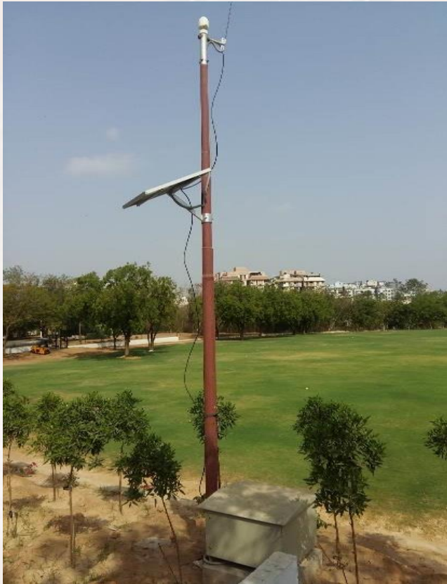
PL Pole at Site
