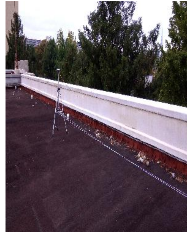
Temporary base station
