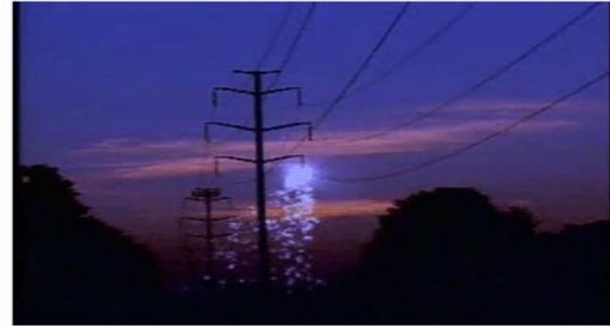
Damage to power grids.
