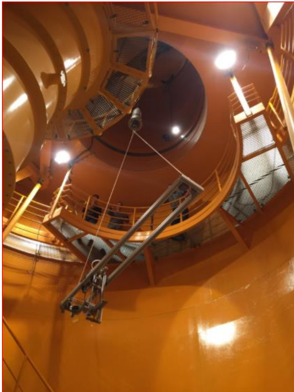
Figure 5-5 Mounting the ERS on the handrail of deceleration chamber – on the right picture the secure mesh and the secure “pillow” are visible
