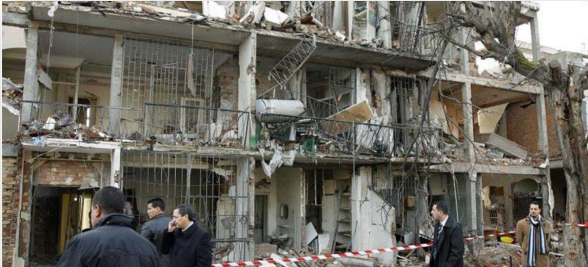
UN Photo/Evan Schneider | A building damaged by the 11 December 2007 terrorist attack across the street from the UN Headquarters complex in Algiers. The bombing claimed the lives of 17 United Nations workers.
