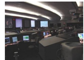
2 Operational Control Centers
