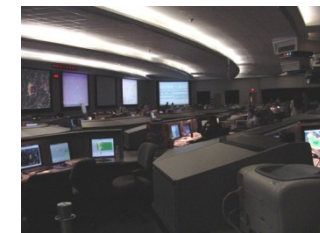
2 Operational Control Centers
