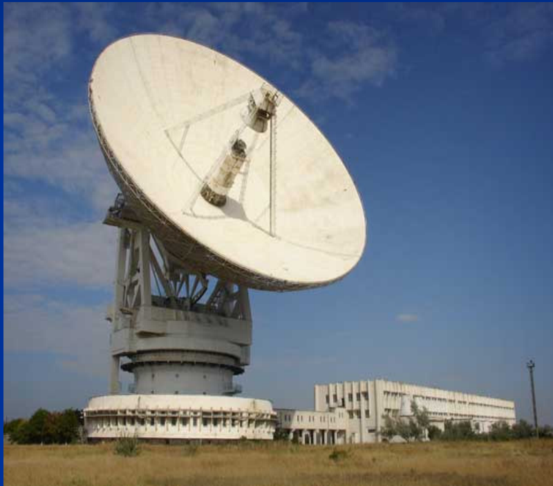
Transmitting telescope RT-70 in Evpatoria
