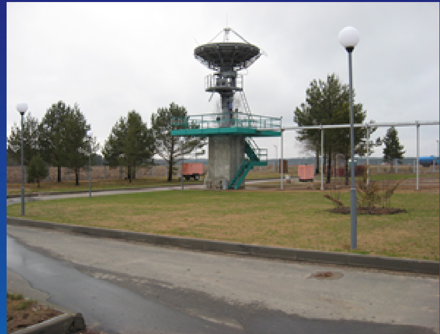
Antenna system of Command- Measuring Station
