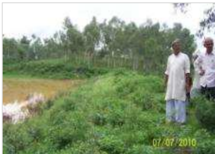
Check dam for in-situ moisture conservation
