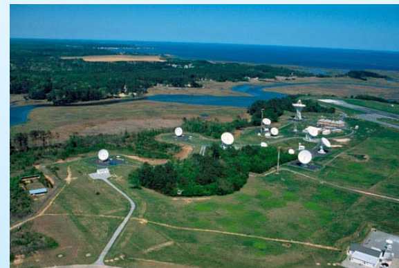
Wallops Command, Data, and Acquisition Station
