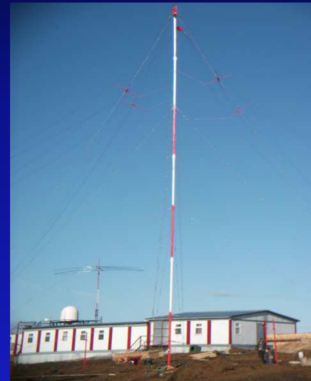
Installation of antenna and feeder complex vertical radio sounding of ionosphere situated on Kheysa island, Franz Josef Land
