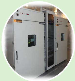
IRNSS Network Timing Facility (IRNWT),Bylalu
