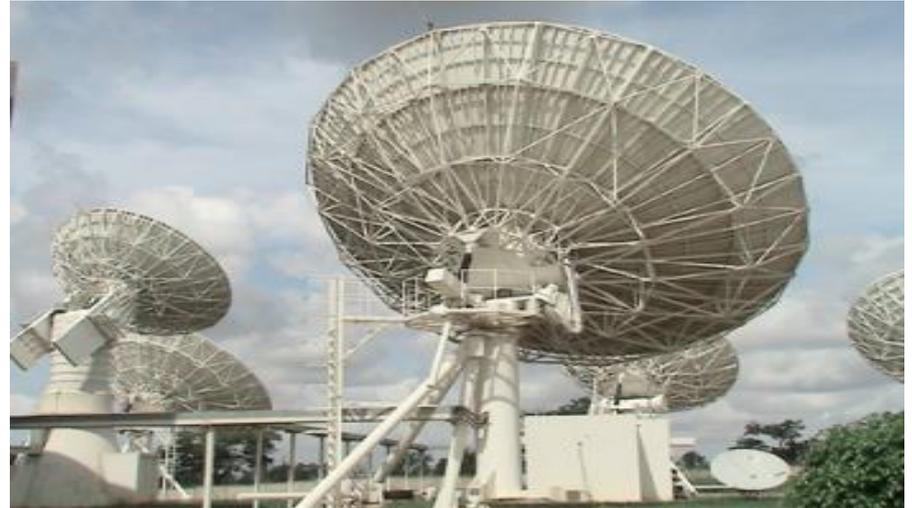
**NIGCOMSAT Master Control Station with C-L Band Antenna Systems**
