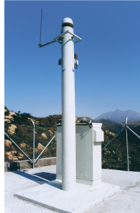
Permanent GNSS Reference Station
