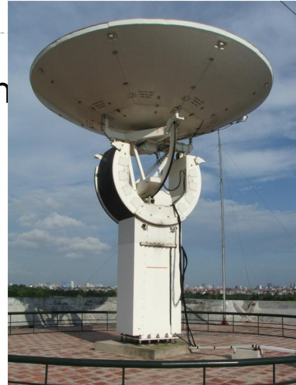
Function: capture image data (SPOT 2, 4, 5 and Envisat ASAR and MERIS), process to produce image products of level 0, 1 and 2, archive them and automatically update the image catalogue.
