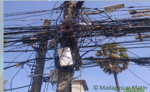
Frequent illegal electricity connections
