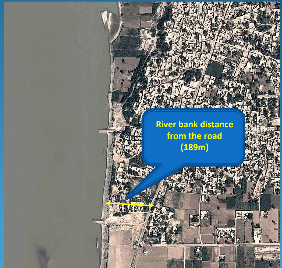
Chashma Barrage Downstream - 2011
