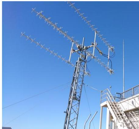
Yagi-Antenna for VHF-band
