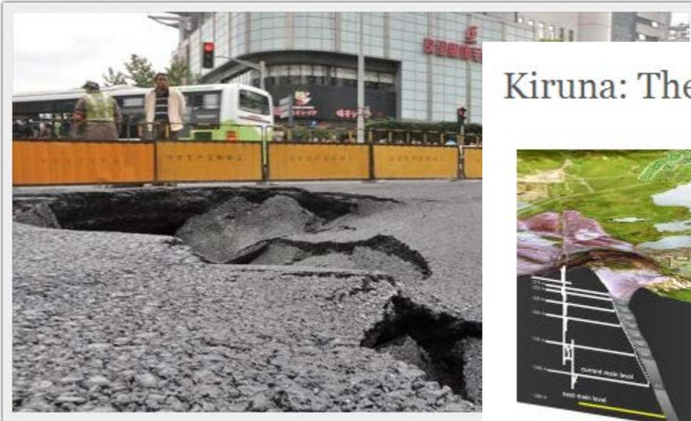
This hole appeared near Shanghai Railway Station to have been caused by subsidence because of moving underground water table. Photo: Cai Xianmin/GT
