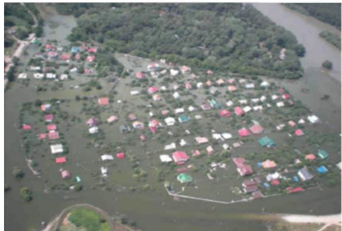
Fig. 1. Flood damage of Nester river (July 2008)
