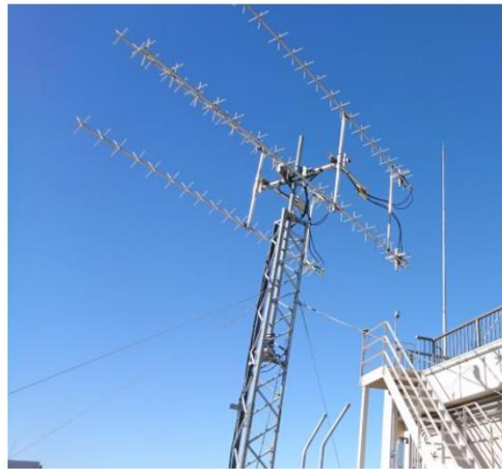
Yagi-Antenna for VHF-band
