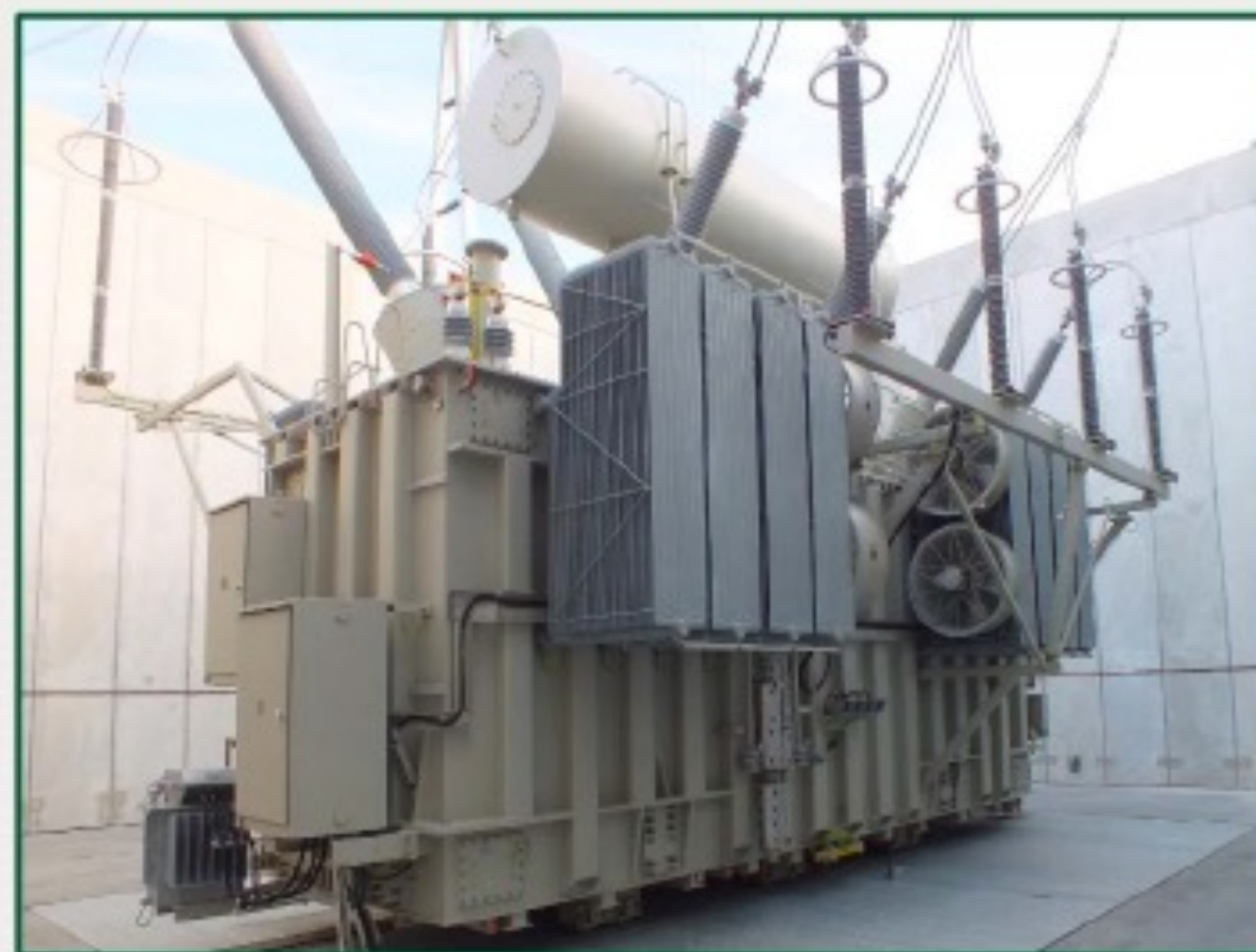
200MVA Transformer (420/66 kV)
