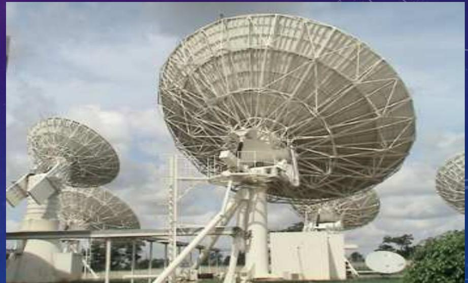
NIGCOMSAT Master Control Station with C-L Band Antenna Systems
