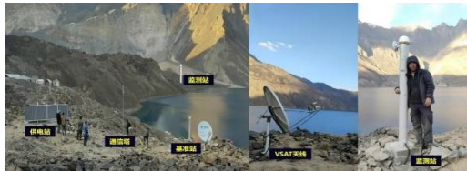
Deformation Monitoring High accuracy Safeguarding for the dam in Sarez Lake
