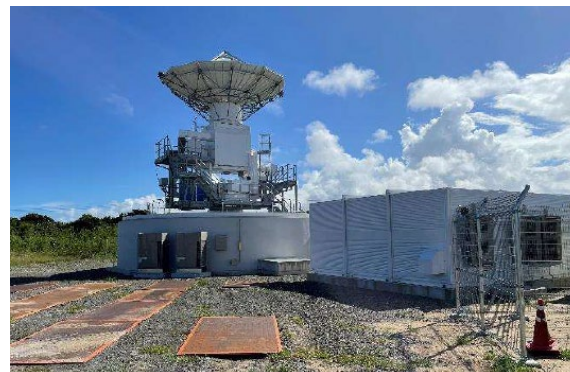
The new TT&C station at Tanegashima-island (Photo taken during construction)
