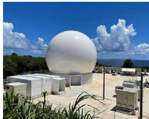
The new TT&C station at Miyakojima-island
