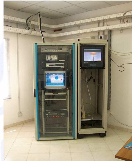
The L-band system hosted at BSC Remote Sensing Centre, used to acquire NOAA/AVHRR and SeaStar/SeaWiFS
