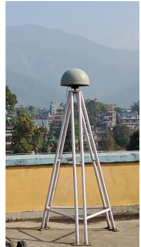
GNSS CORS Antenna at Western Region Campus, IOE Tribhuvan University Pokhara
