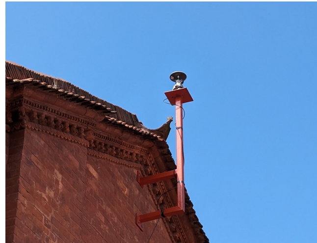
Low-cost GNSS CORS at Khowpa College of Engineering, Tribhuvan University Bhaktapur
