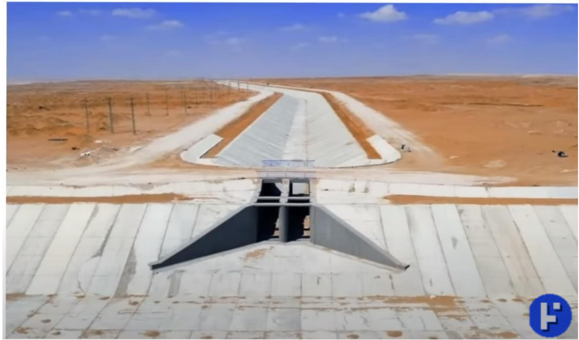
Underground pipes transporting agriculture wastewater from the Rosetta branch to a new artificial river
