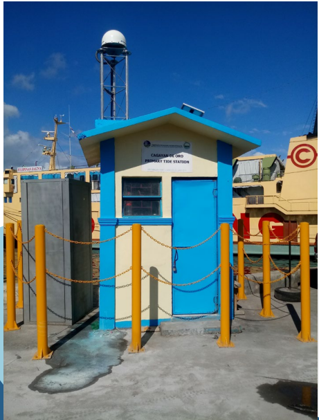
OTT Tide Gauge and GNSS Receiver.
