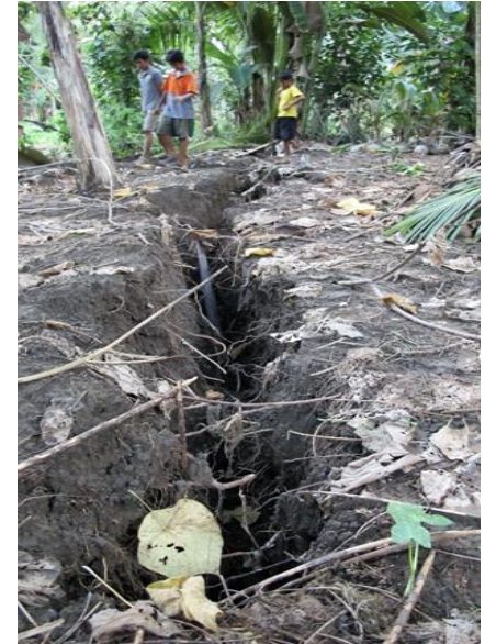
Lateral spread that appeared in Brgy. Tamlangon after the M6.6 earthquake that has worsened after the M6.5 earthquake
