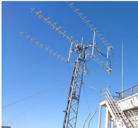
Yagi-Antenna for VHF-band
