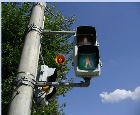
Traffic lights with sound signal system
