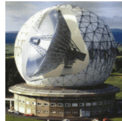
TIRA Radar / FGAN, Germany 2cm \phi at 1000km [2]
